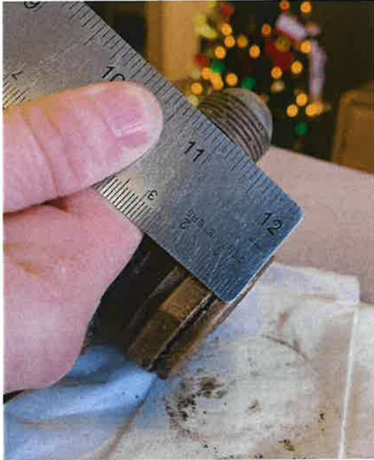
Measurement of base corrosion.
