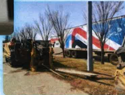
Fiber Optic Deployment
